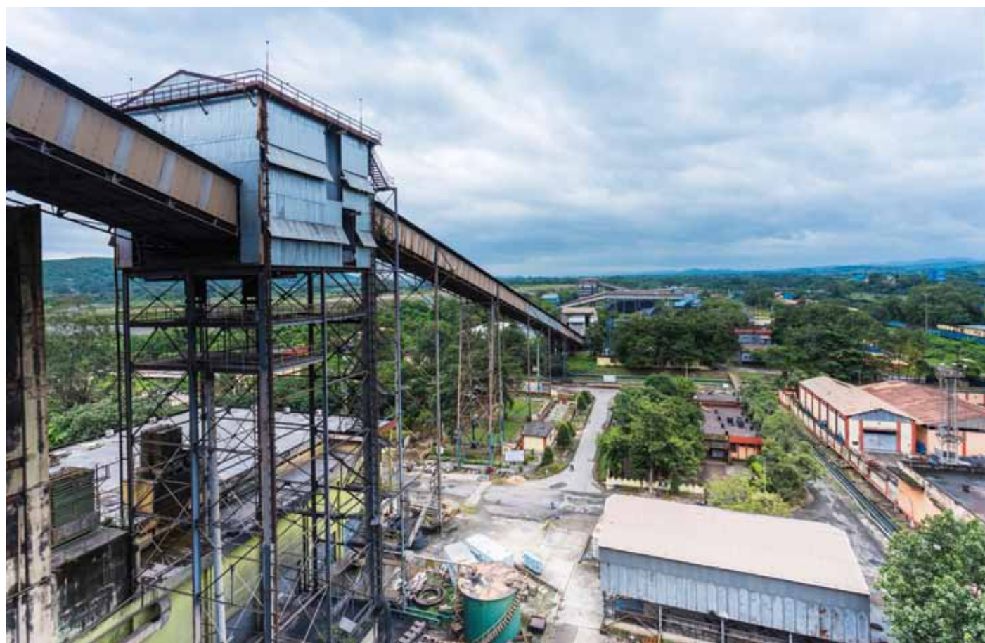
CHP Coal Handling Plant Area, Rourkela
