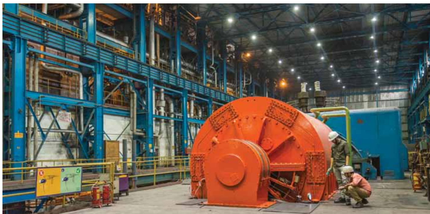
PP-II TG Hall, Durgapur
